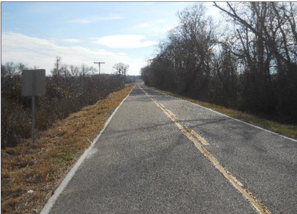
Photo 6: View Looking South From Bridge
