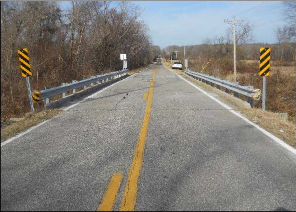
Photo 4: Northbound Bridge Approach
