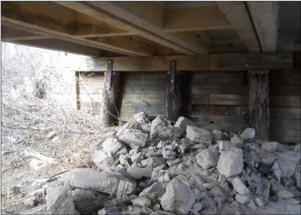
Photo 10: North Abutment Of Bridge
