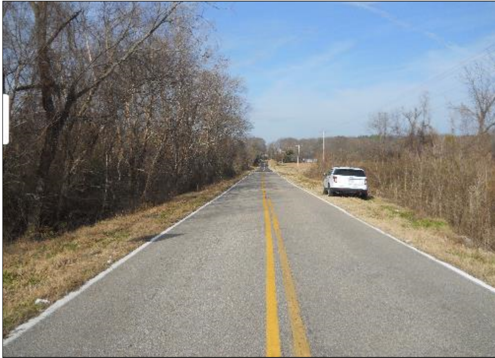
Photo 5: View Looking North From Bridge
