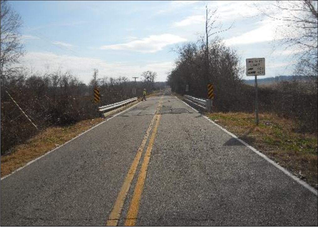
Photo 3: Southbound Bridge Approach
