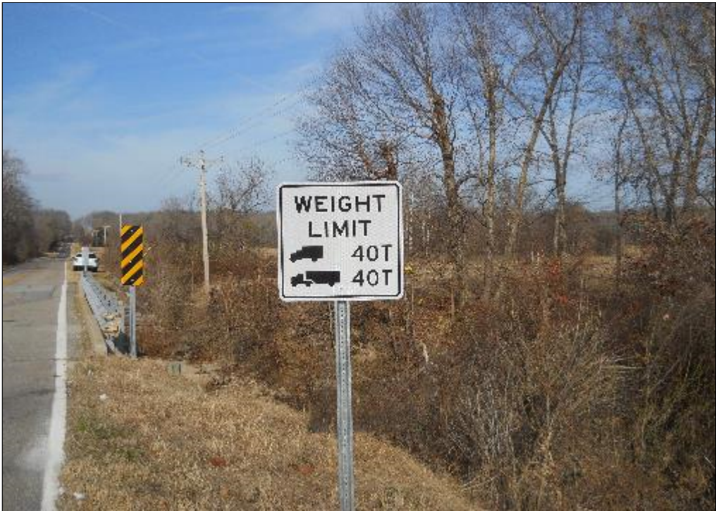
Photo 2: Bridge Load Rating
