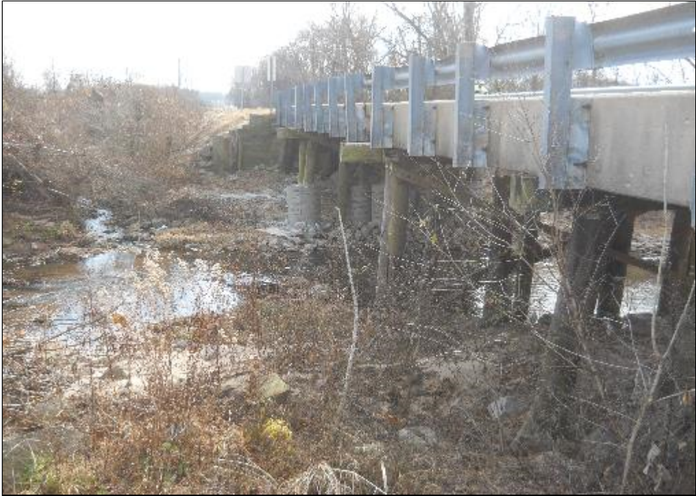
Photo 9: Upstream Profile View Of Bridge
